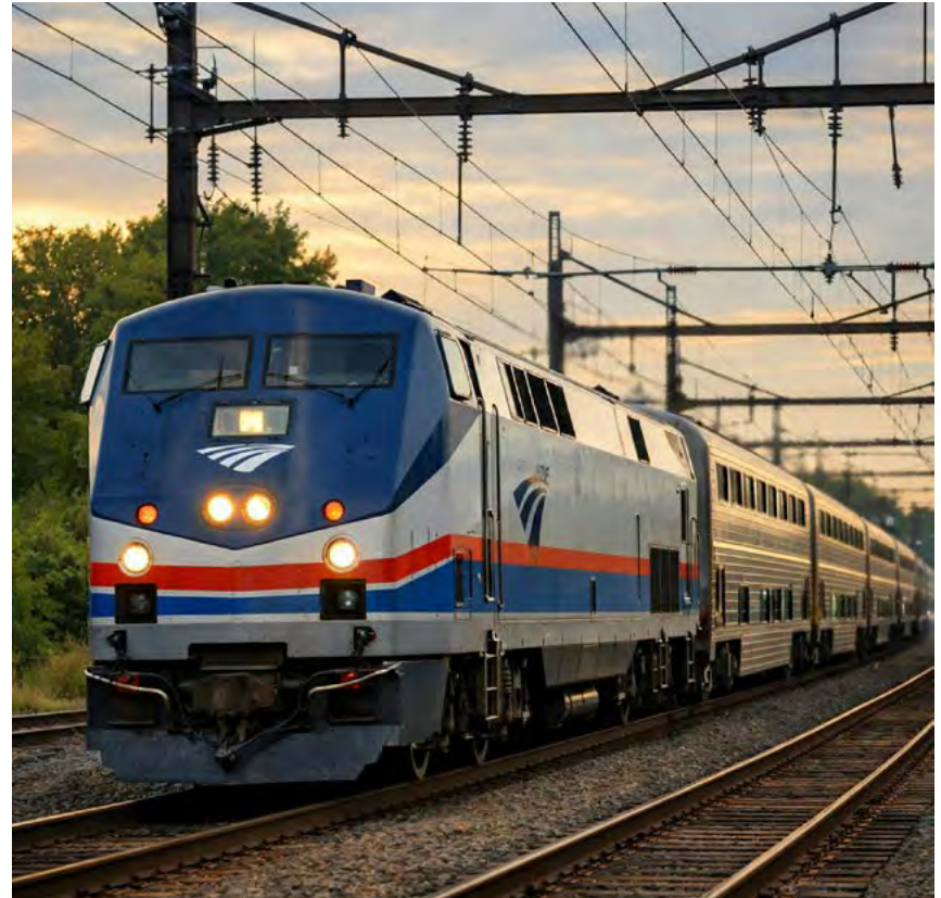
PennDOT works closely with Amtrak to improve stations and relocate overhead arched cable systems in southeast Pa.
