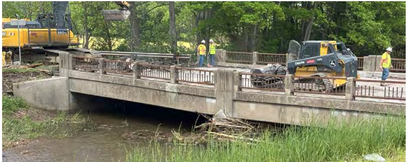
On May 16, 2025, two days after the bridge was closed, demolition began on the 102-year-old bridge.
