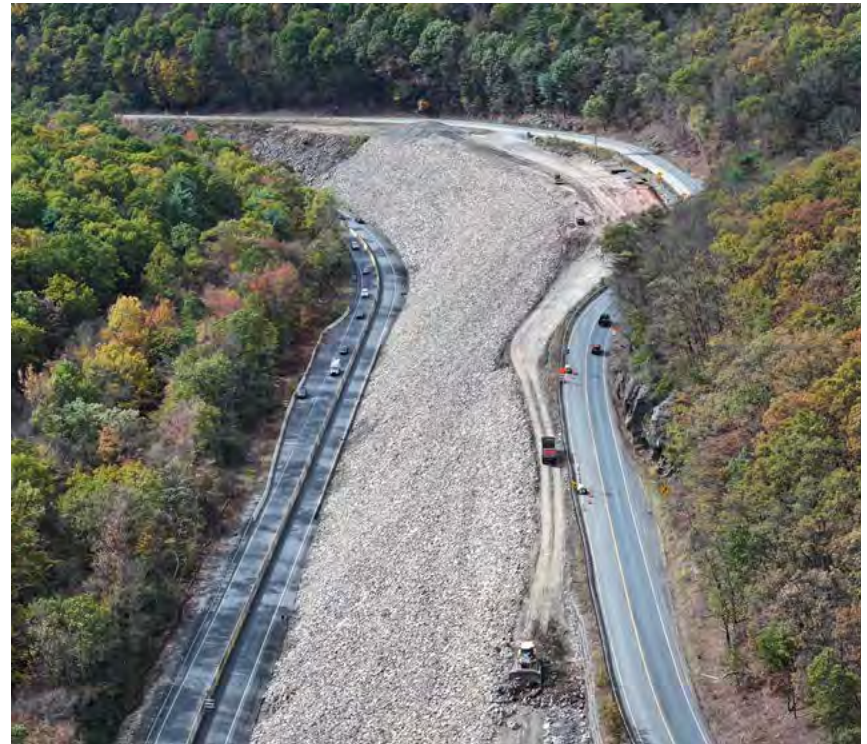
Route 61 widening and curve realignment construction.
