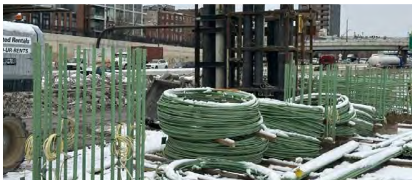
I-95 CAP Project surface level utility work.
