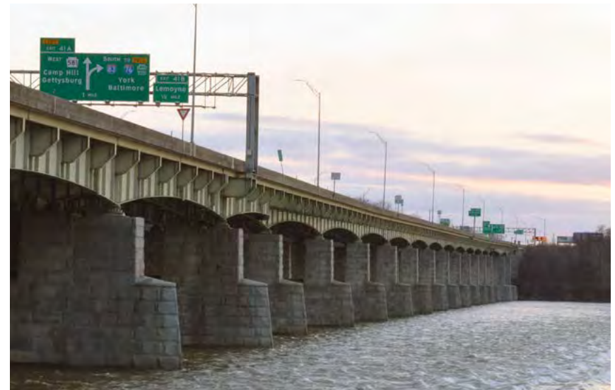
Interstate 83 John Harris Memorial (South) Bridge.
