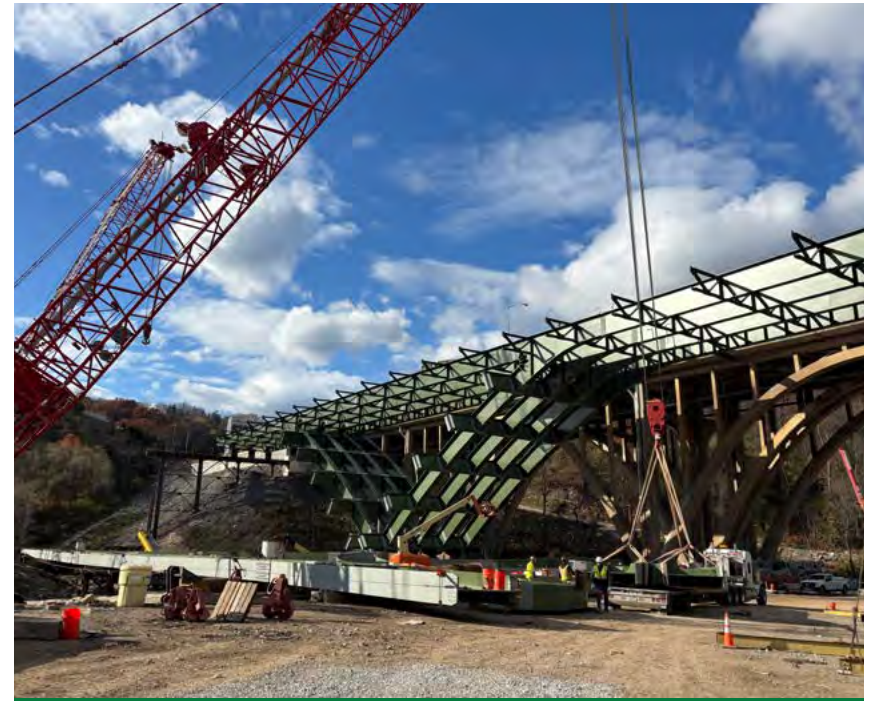
I-376 Parkway East Commercial Street Bridge Accelerated Bridge Construction.
