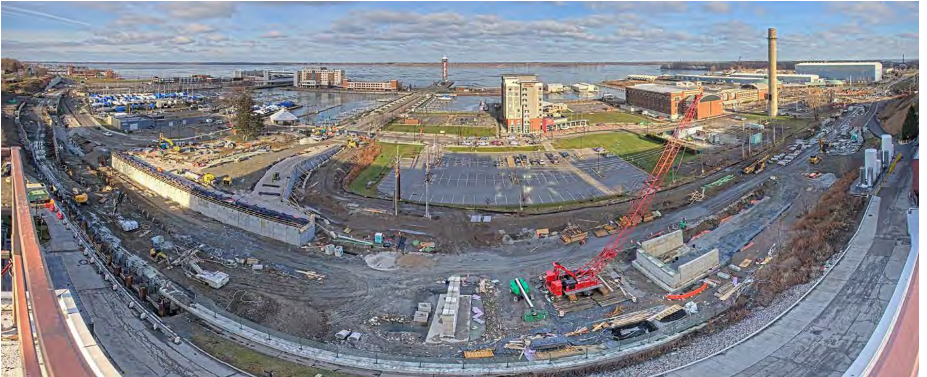
Bayfront Parkway Improvement Project construction in Erie, Pa.
